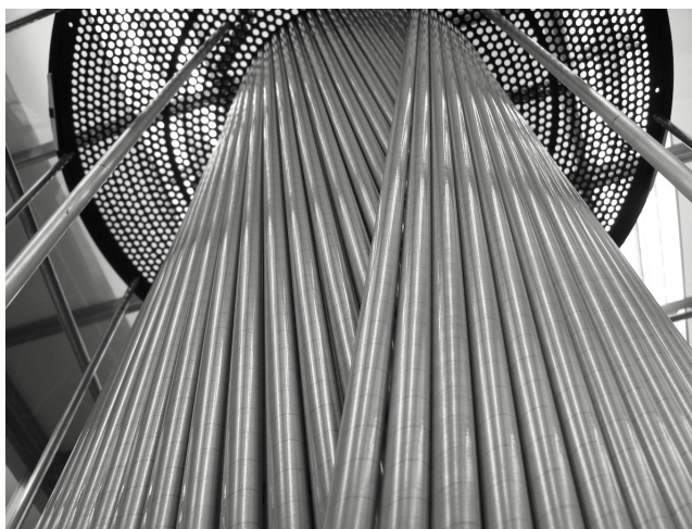
Figure 15: The Central Drift Chamber during construction. A partially completed layer of stereo straw tubes is shown, surrounding a layer of straw tubes at the opposite stereo angle. Part of the carbon fiber endplate, two temporary tension rods and some of the 12 permanent support rods linking the two endplates can also be seen.
